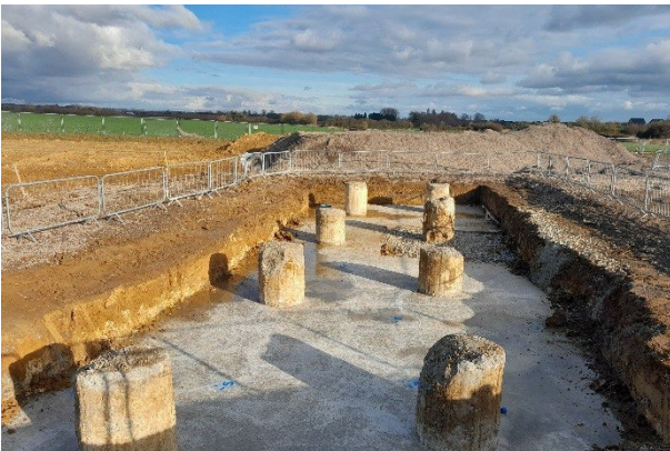
Figure 3: North Abutment dug down and blinded.
