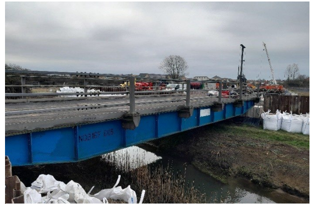
Figure 4: Temporary Bridge over Black Ditch
