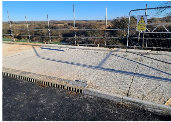
Image 6 - Concrete infills on viaduct
