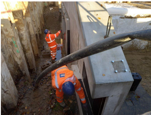
Image 1 Culvert units being installed
