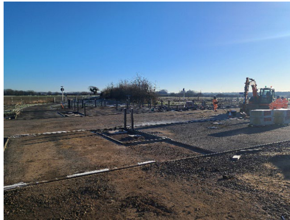
Image 4 - Pegasus crossing and fencing beams
