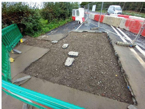
Image 3 Complete water diversion
