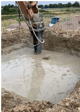
Image 7 Deep Soil mixing
