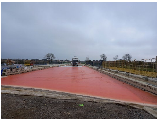
Image 6 waterproofing on the viaduct
