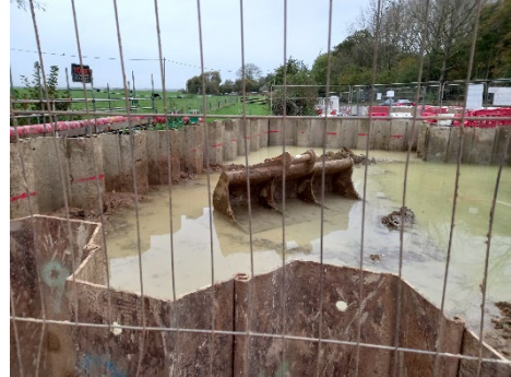
Image 4 Soil improvement completed
