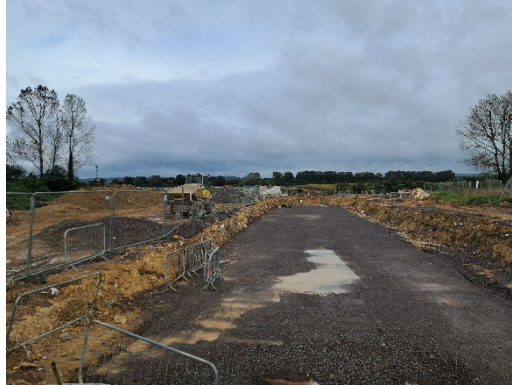
Image 7 Continued Attenuation tank works
