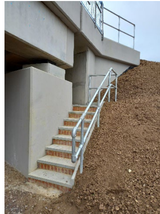
Image 7 North abutment stairs
