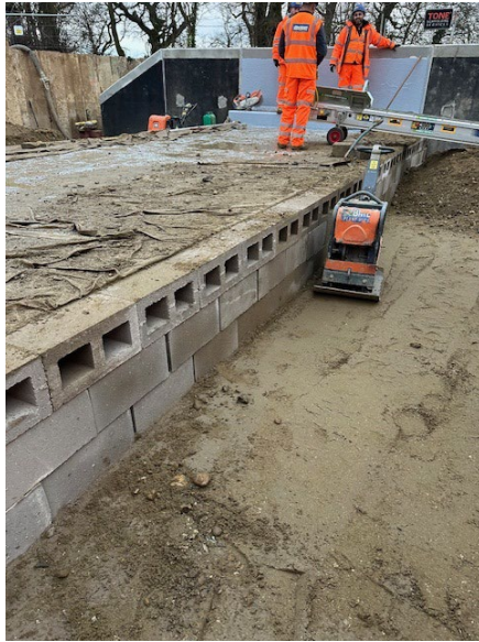
Image 1 - 6n Backfilled and hollow blocks installed
