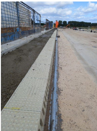
Image 5 Drainage on the viaduct
