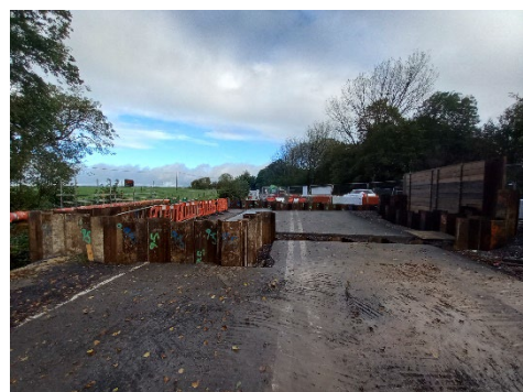
Image 2 Cofferdam installed
