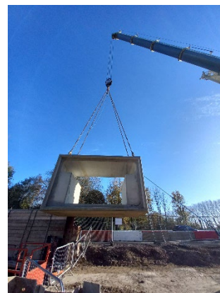
Image 2 Crane lifting precast units
