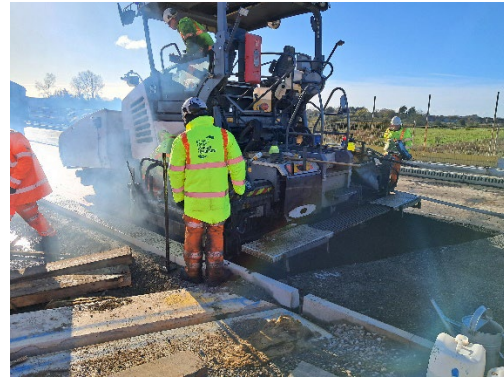
Image 7 Tarmac getting laid on the viaduct
