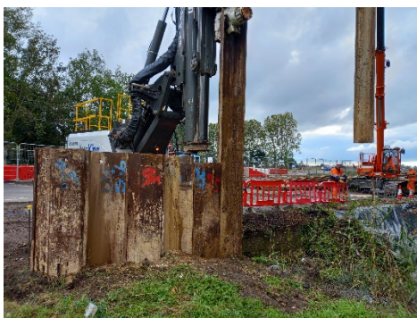
Image 1 Sheet piles being installed
