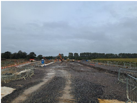
Image 5 Embankment and drainage works
