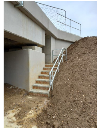
Image 9 South Abutment stairs
