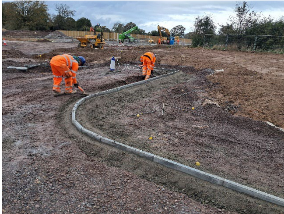
Image 6 Embankment and drainage works
