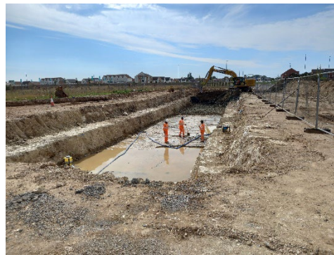
Image 8 Digging out for Attenuation tank
