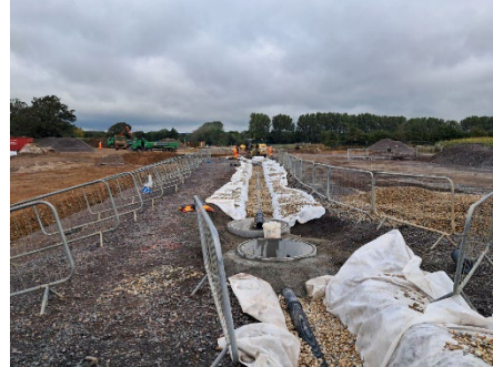
Image 6 Embankment and drainage works
