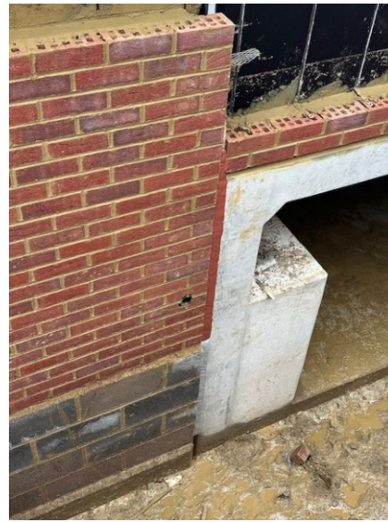
Image 2 - Brickwork on face of culvert
