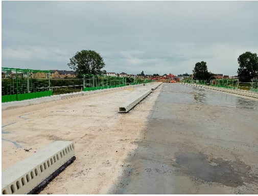
Image 6 Drainage kerbs on viaduct
