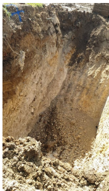
Image 8 Excavation for soil mixing.
