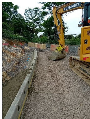
Image 4 Link road kerbs.
