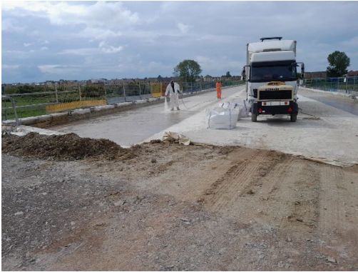
Image 6 Water proofing of the viaduct.
