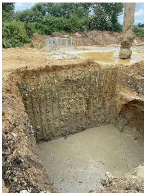
Image 8 Excavation ready for mixing
