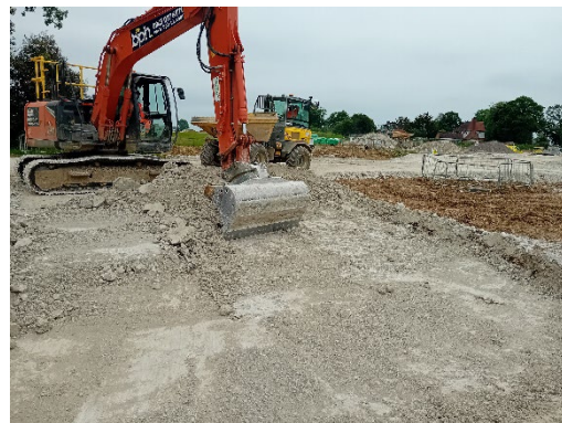
Image 2 Access track from chalk level.
