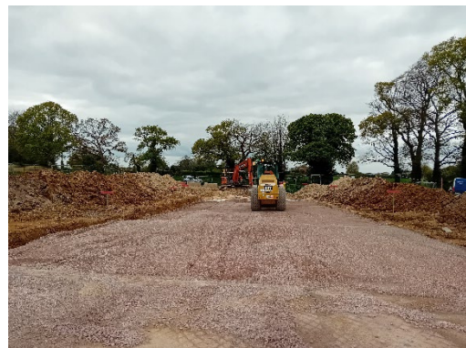
Image 5 Link road with type 1 aggregate.
