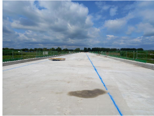
Image 7 Concrete deck of viaduct.
