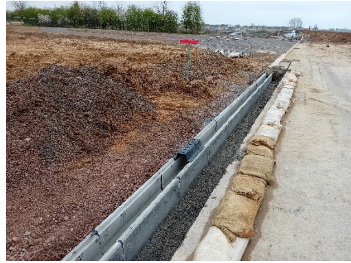
Image 4 Channel drains.
