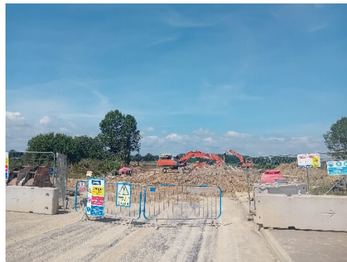
Image 9 Soil mixing at south side of site
