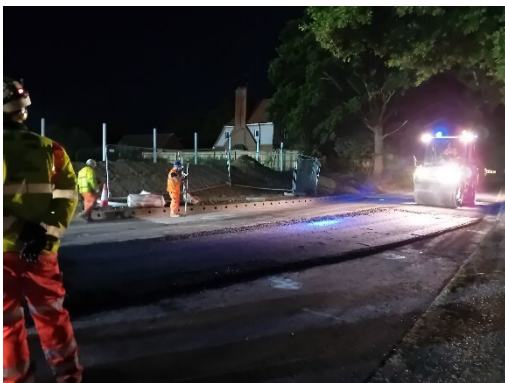
Image 4 Tarmac tie-in on link road
