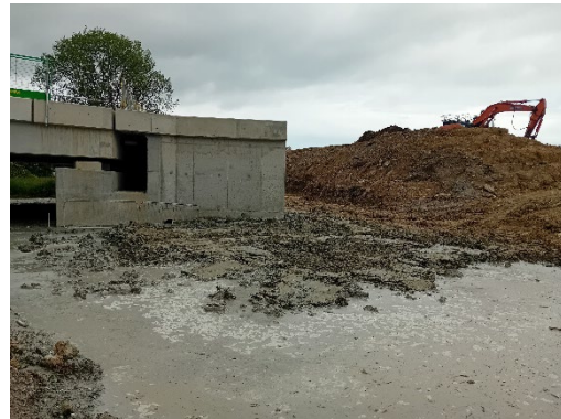
Image 9 Soil mixing around South end.
