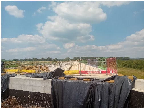
Image 8 South of viaduct.
