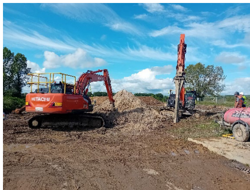
Image 9 Soil mixing machines at the southern end of site.
