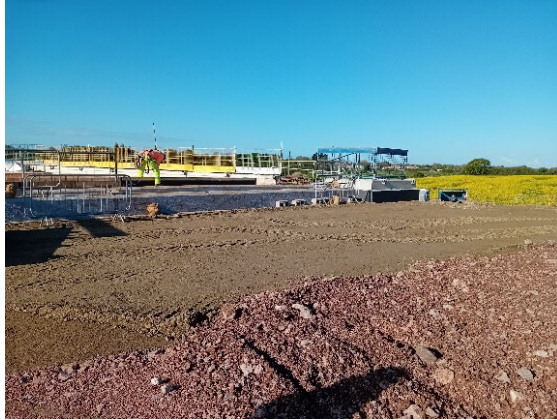
Image 6 Northern end of the viaduct
