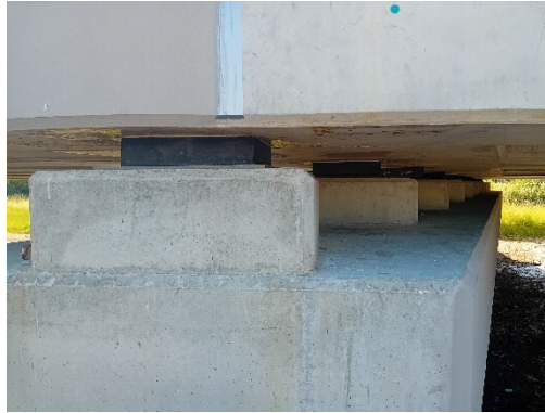
Image 7 Bearing between viaduct deck and pier.
