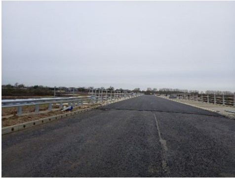
Image 6 – Parapet tying into VRS
