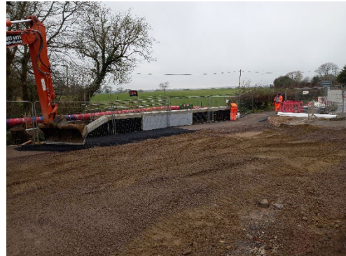
Image 2 – Temporary footpath installation
