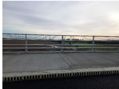
Image 5 – Parapet works on viaduct
