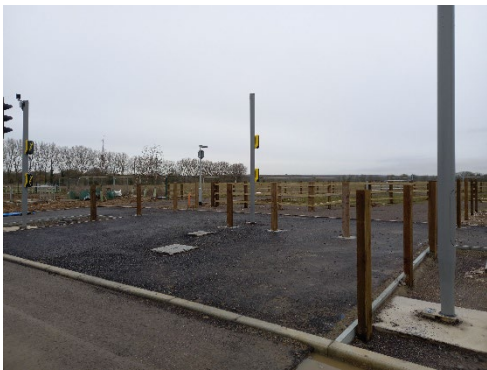
Image 4 - Pegasus crossing and fencing beams
