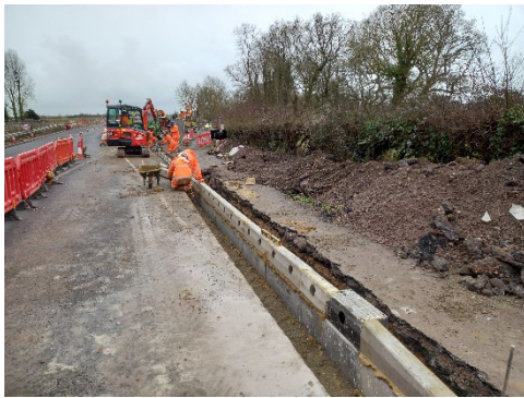
Image 1 – Kerb installation
