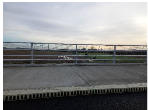
Figure 6 - Parapet and mesh panels
