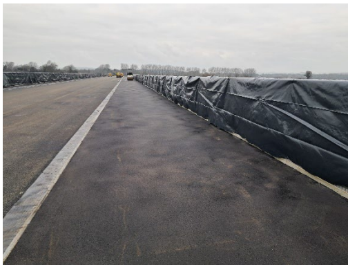
Figure 5 - Surface course on footpath
