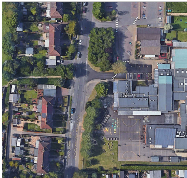
NORTH SOUTH AERIAL VIEW
