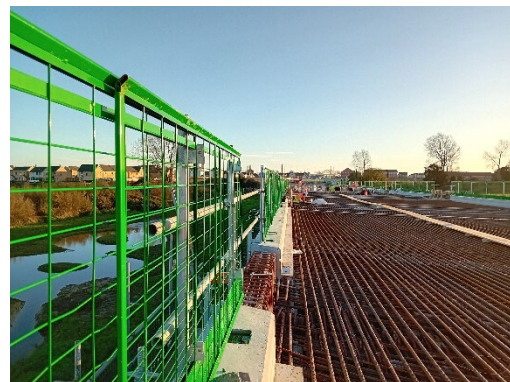
Image 6 Final parapet ready for concrete.
