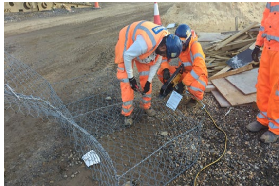
Image 6 Gabion basket being made for Southern swale
