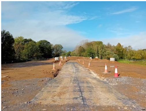
Image 1 Track mats placed running up to surcharge
