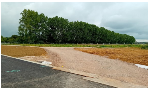
Image 1 Access track for northern pond.
