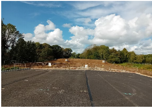
Image 2 Embankment with surcharge.
