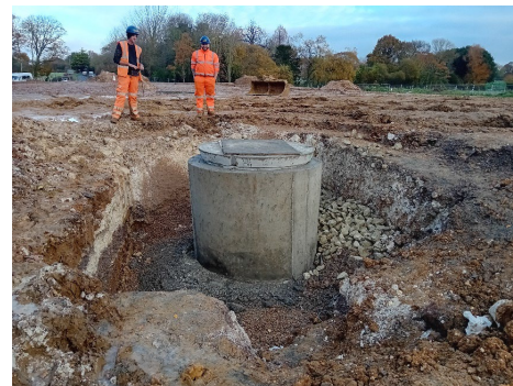
Image 2 Manhole for drainage.
