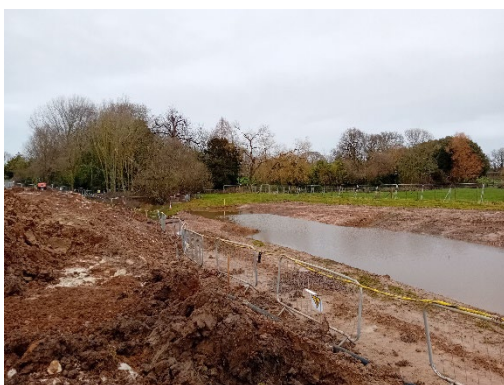
Image 1 Newly dug swale.
