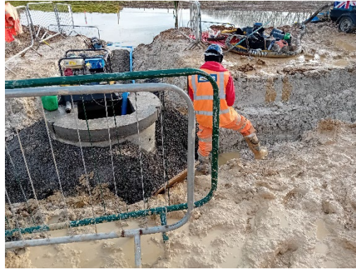
Image 3 Continued drainage works.
