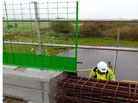
Image 9 Steel work on parapet wall.
