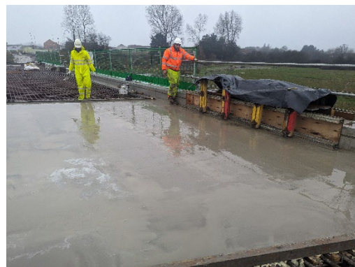
Image 9 Fresh concrete pour.
