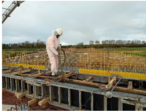
Image 7 North abutment concrete pour.
