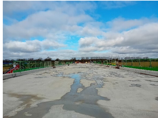
Image 7 Concrete deck on viaduct.
