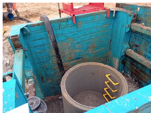
Image 2 Water pump in manhole trench box.
