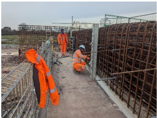
Image 5 North abutment reinforcement.
