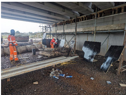
Image 8 Shutters ready for instalment.
