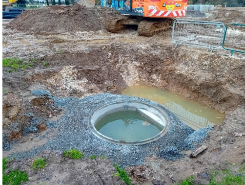
Image 4 Manhole draining northern pond.
