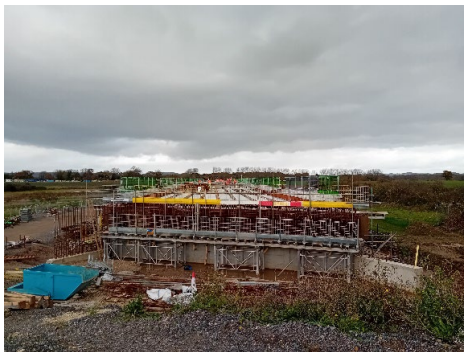
Image 8 Bridge progress facing North.
