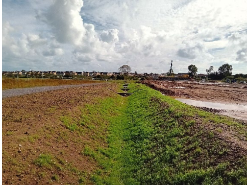
Image 3 Swale for storm drainage.
