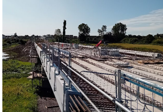
Image 4 Beams in position.
