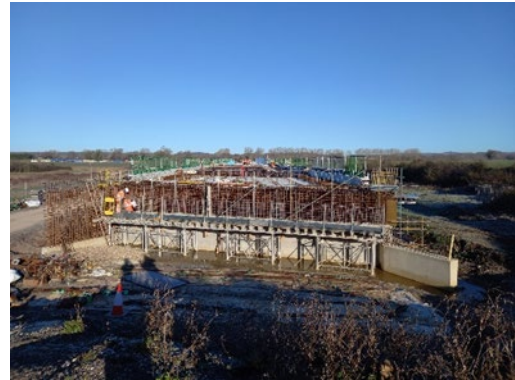
Image 8 View of viaduct facing North.
