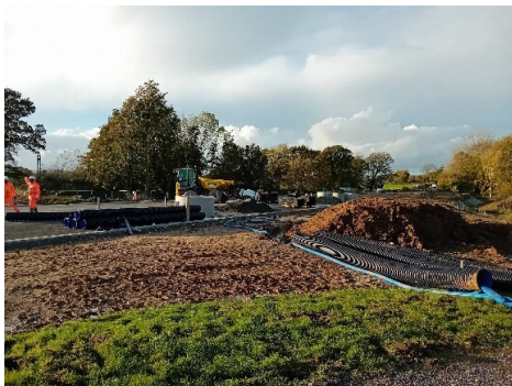
Image 1 Drainage pipes and pumping out ground water.
