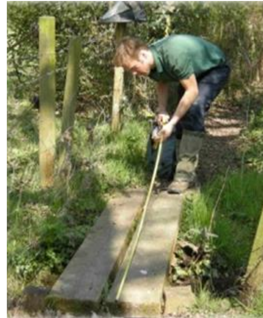
Access Ranger measuring a plank bridge while inspecting a parish
