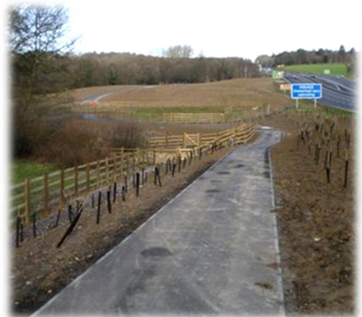
The new bridleway by the A23
