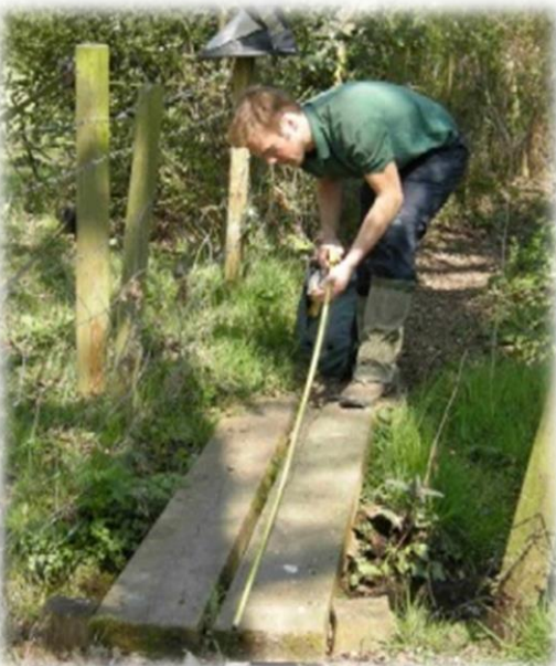
Measuring a bridge to be replaced
