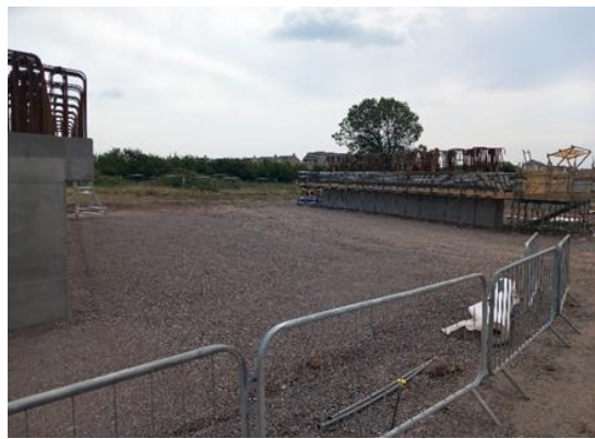
Image 7: Area between piers tidied and scaffolding put up
