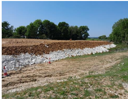
Image 1: Chalk embankment being surcharged
