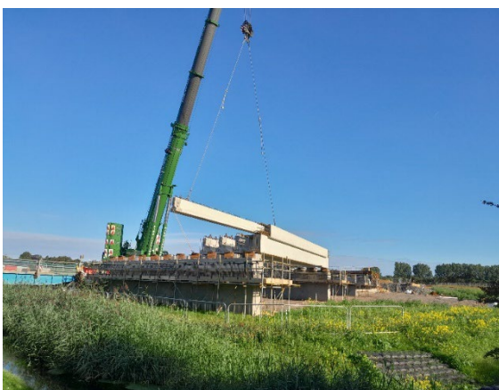
Image 4: Beams being lifted into position
