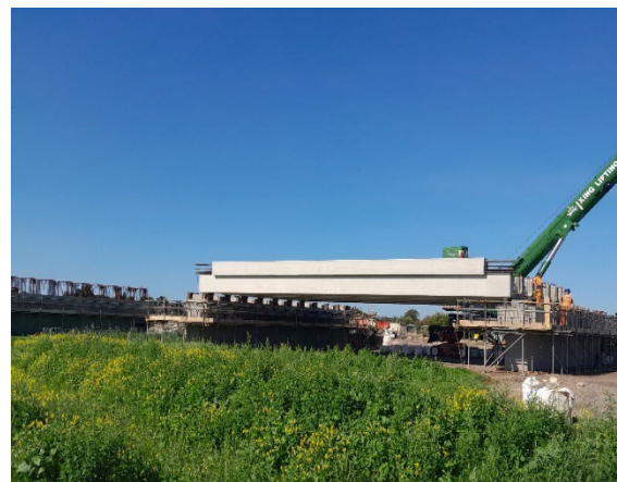
Image 5: The beams in position
