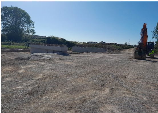
Image 6: Crane mat construction
