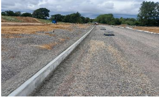
Image 2: Kerbing along northbound carriageway
