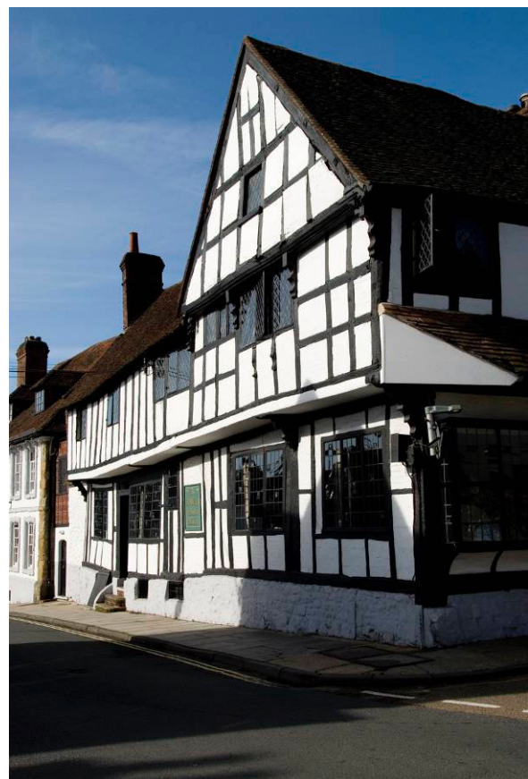
Fig. 7. The Spread Eagle Hotel, South Street.
