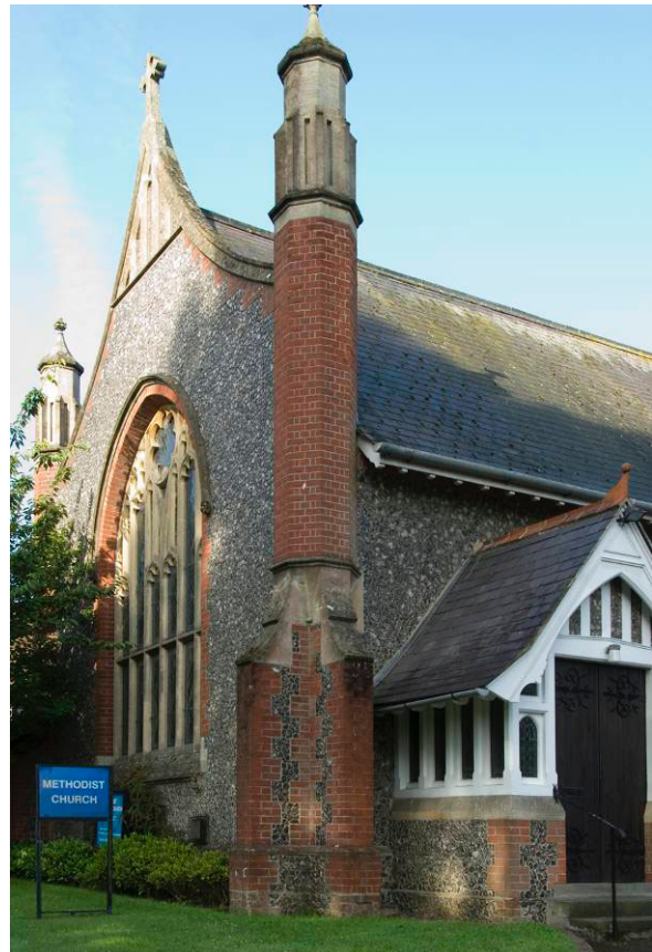
Fig. 10. Methodist church, North Street.
