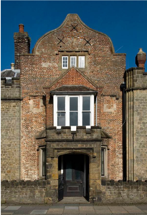
Fig. 18. Capron House, North Street.
