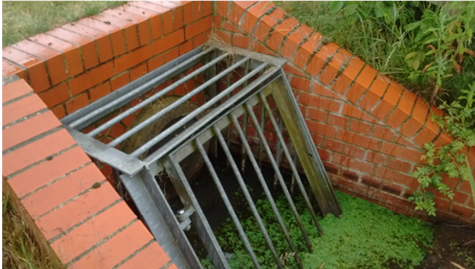
Figure 1-Culvert with Wingwalls and Trash Screen
