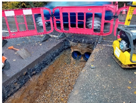
Image 3 Drainage for culvert into Brookfield stream.
