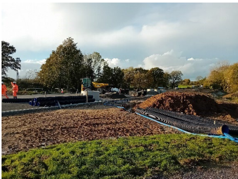
Image 1 Drainage pipes and pumping out ground water.
