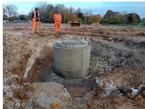
Image 2 Manhole for drainage.
