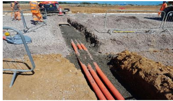
Image 3: Duct crossing beneath the road
