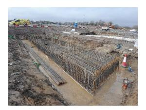
All the piers North of Black Ditch has been dug to the correct levels and blinded. Blinding is non-structural concrete that is there to provide a clean and level working area. This week, steel fixers have arrived on site to start constructing the pile caps. A pile cap is a thick concrete mat that will evenly distribute the loads from the viaduct into the piles.
