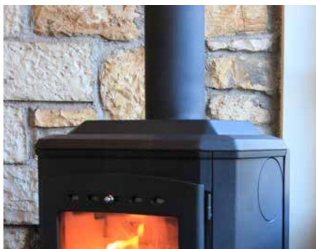
The firebox can be managed to ensure that the flue gas temperature is not excessive (approx 200 degrees C) at the level of the thatch.
