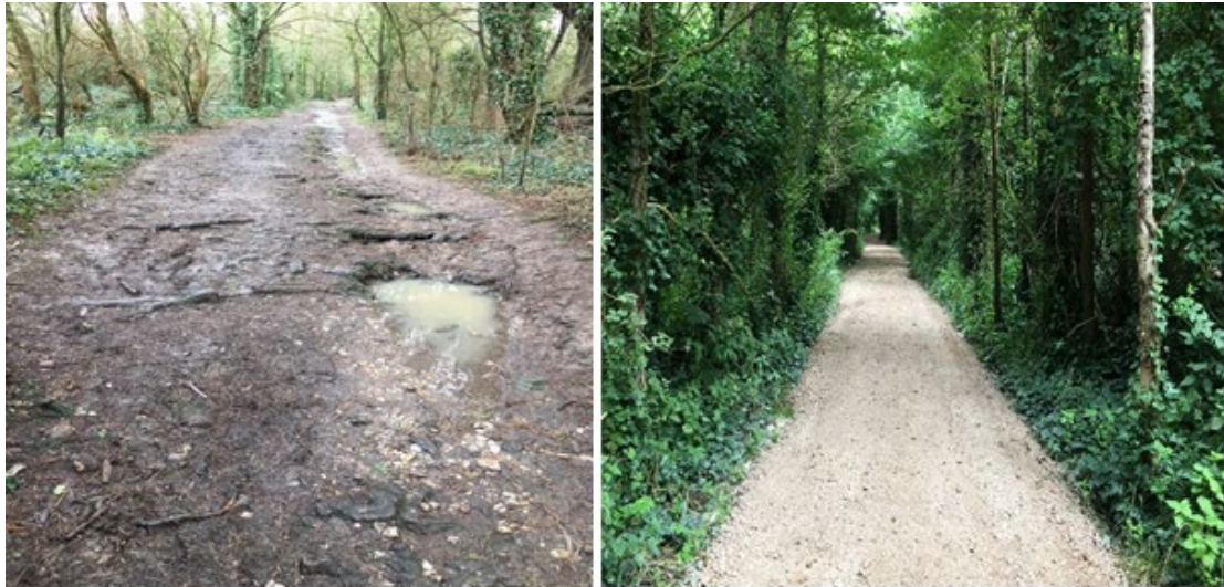
Surfacing improvement works along Cow Lane, Angmering, undertaken using S106 funds
