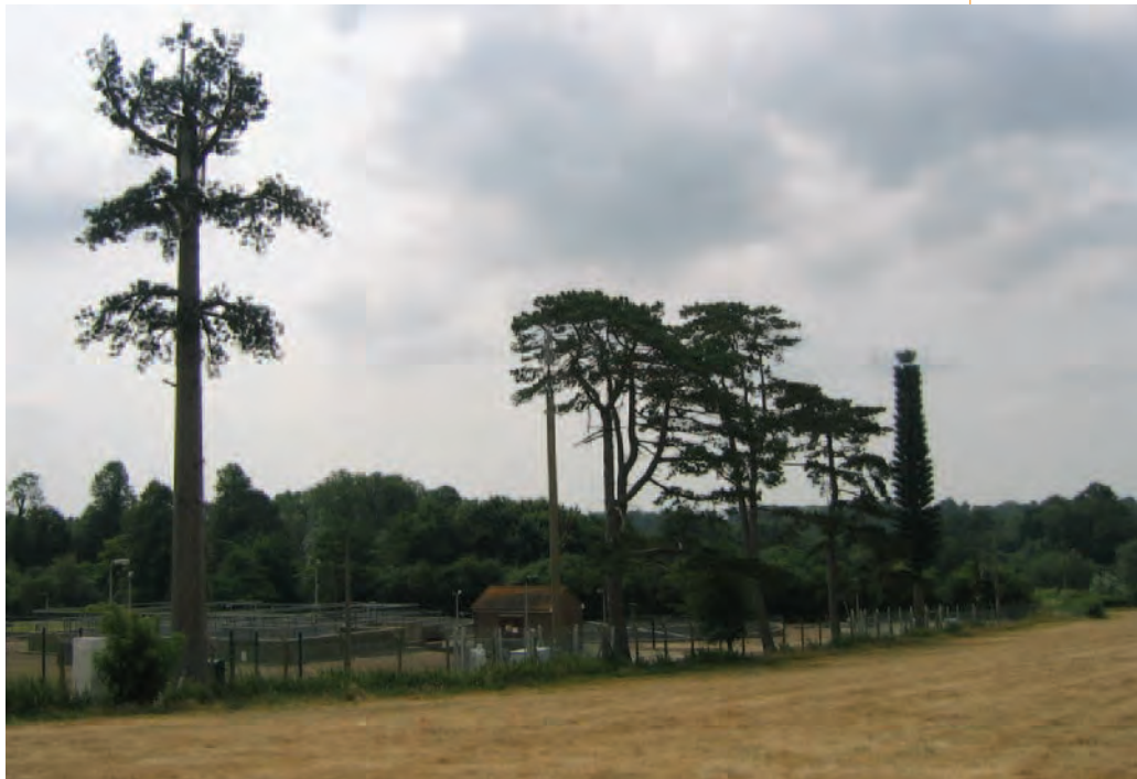
Disguised telecommunication masts near Cuckfield
