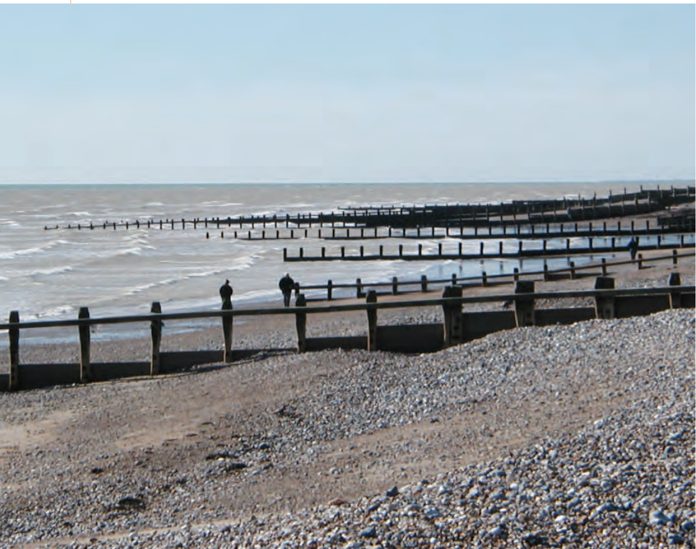
Groynes along the shingle beaches of the West Sussex coastline
