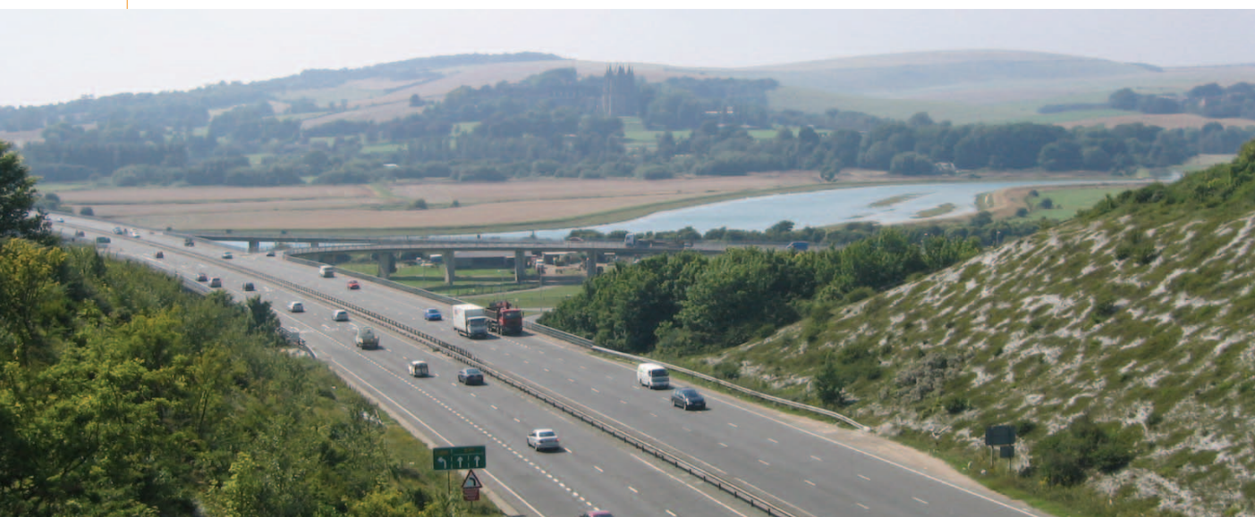
The A27 Trunk Road crossing of the River Adur near Lancing College, Shoreham-by-Sea
