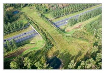
Figure 10. 'Eco-aqueduct' over 'sunken' motorway on the new A4 in Holland (Google)
